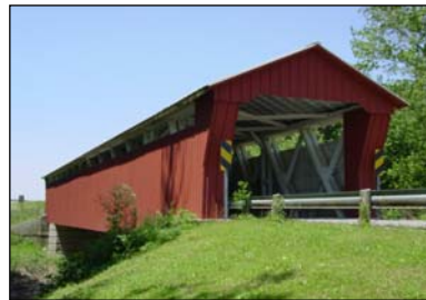
McColly Covered Bridge 13-1.56 over the Great Miami River
